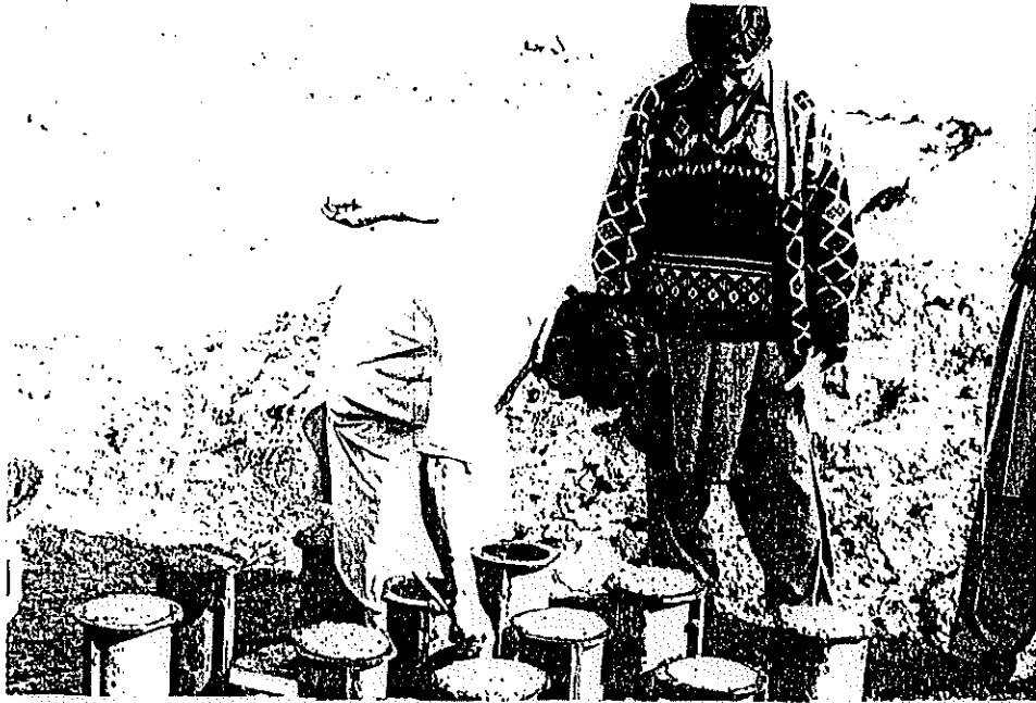
Photo - 23 Concrete being sampled from project by NTRC technicians
